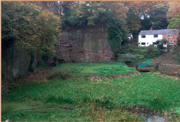
Worsley Delph in 2017 following the clearance of scrub vegetation from The Island at an early stage in the restoration works
