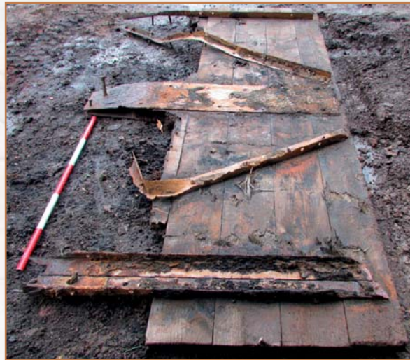
The remains of the sluice gate removed for renovation
