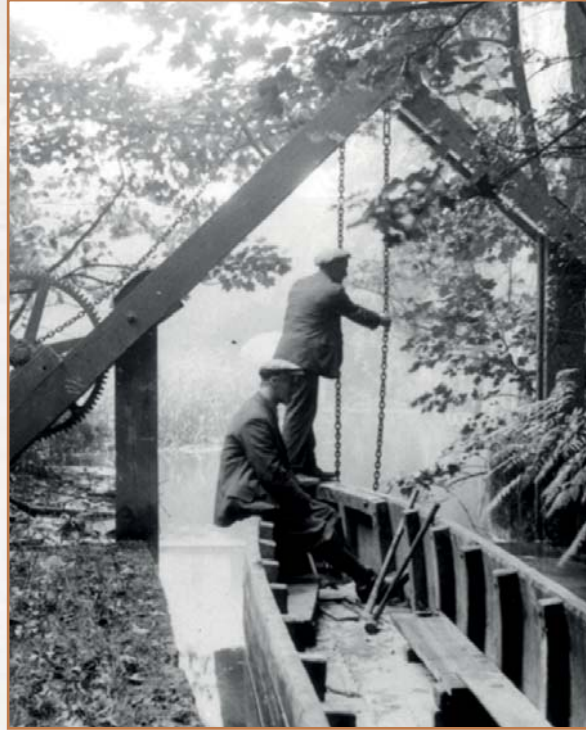
Operating the sluice at the entrance to the western tunnel
