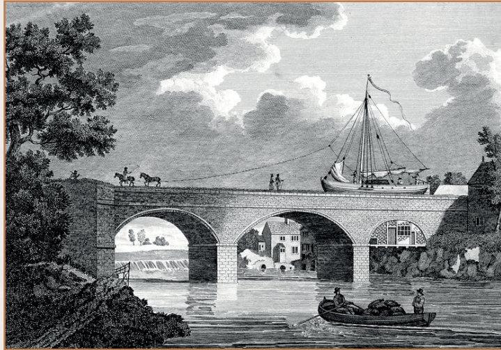
An engraving of c. 1794 featuring James Brindley's remarkable aqueduct carrying the Bridgewater Canal across the River Irwell
