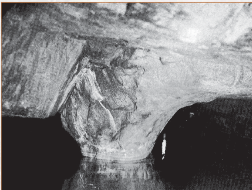
A view of 'Waters Meeting' where the two entrance tunnels converge
