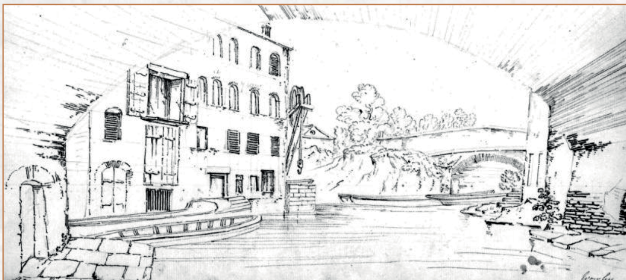
View of the eastern basin through the second arch of Worsley Road Bridge in 1807, showing the Duke's warehouse, the narrow towpath and the doorway into a workshop beneath the adjacent arch
