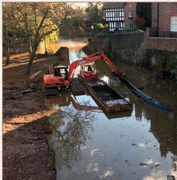
View across the western basin from Worsley Road Bridge in 2018, showing the remains of a sunken boat being exposed during the removal of silt
