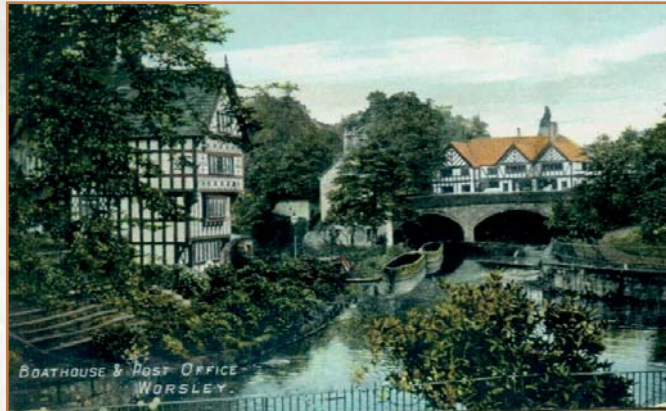
A postcard view taken in 1907, showing the eastern arches of the bridge in front of the half-timbered building that replaced the corn mill in c. 1903
