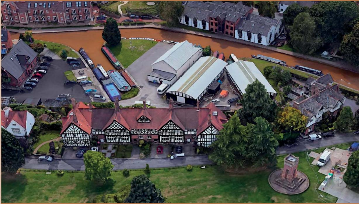
Estate houses and the monument to the 3rd Duke of Bridgewater on The Green
