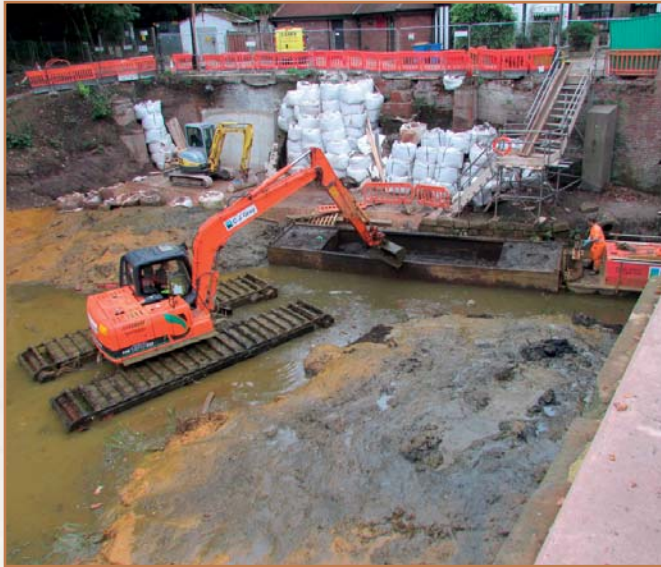
Dredging the canal basin at Worsley Delph in 2018/2004
