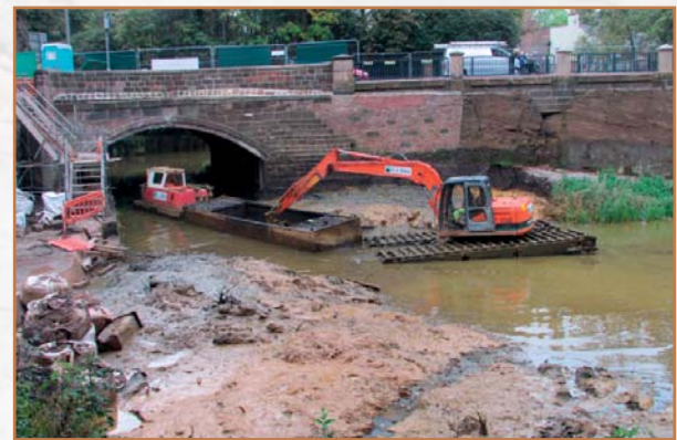
Dredging the canal basin in 2018
