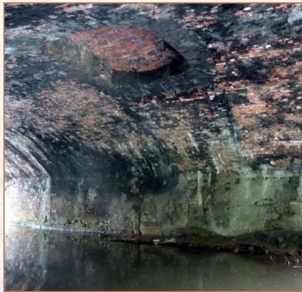
The blocked-up aperture for the hoist in the bridge arch
