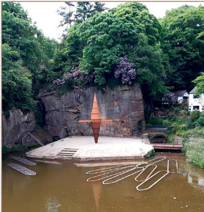
View of Worsley Delph and The Island upon completion of the restoration work
