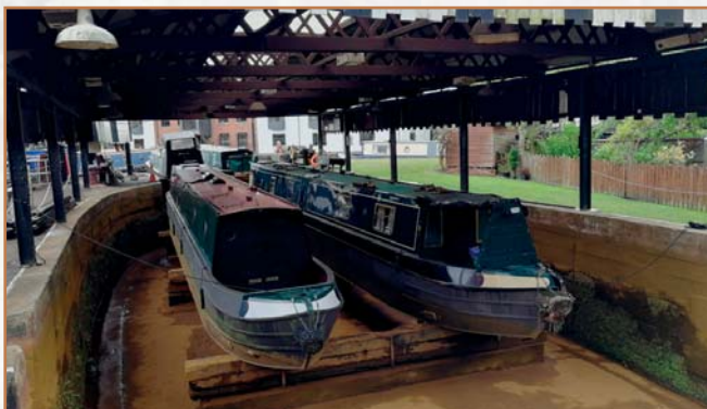
Worsley dry dock continues to be used for boat repairs
