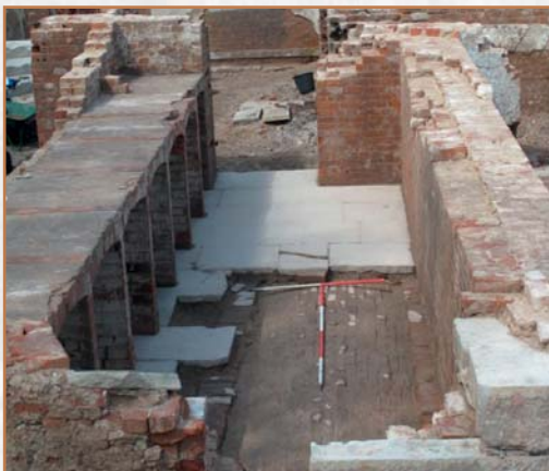
One of the store rooms, showing the top of the brick-vaulted cellar beneath the flagstones
