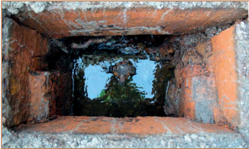
A clack-valve chamber uncovered on The Island
