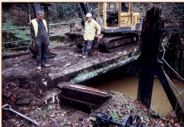
Monitoring the installation of a water-treatment pump in 2004
