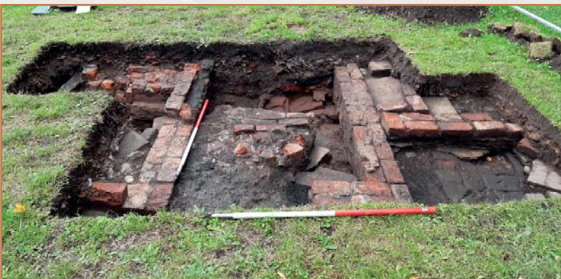
Trench excavated across the outbuildings to the Manor House in 2019 (courtesy of Dr M Nevell)
