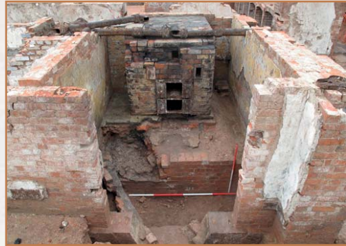
The basement boiler room
