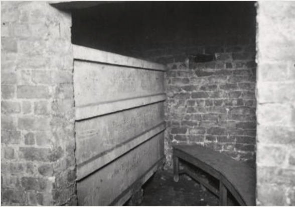
An open vault, photographed in 1906 (copyright Manchester Libraries, Information and Archives, Manchester City Council)
