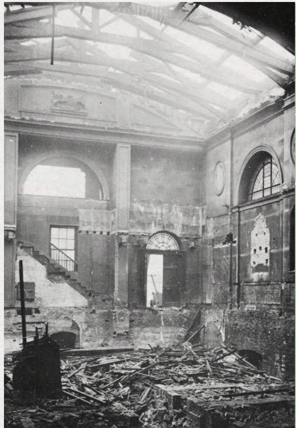
A photograph taken inside during the demolition of St Peter's church in 1907, with the vaults visible below the floor (copyright Manchester Libraries, Information and Archives, Manchester City Council)
