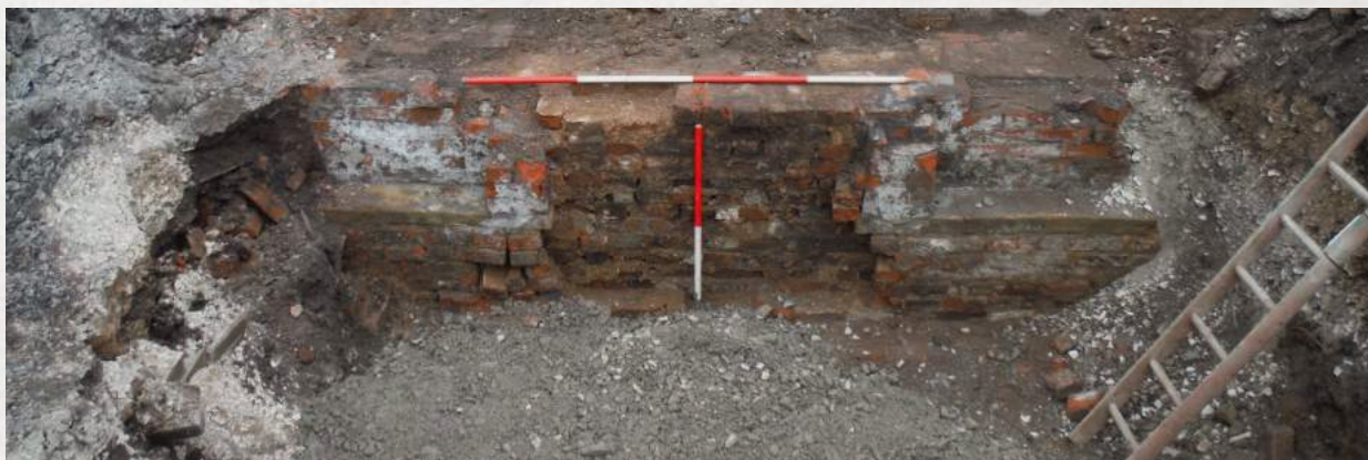
A cellar on the site of the Mosley Street Buildings
