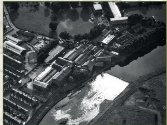
Aerial view of the Irwell Bank Works taken in 1988, shortly before its demolition (courtesy of GMAAS)
