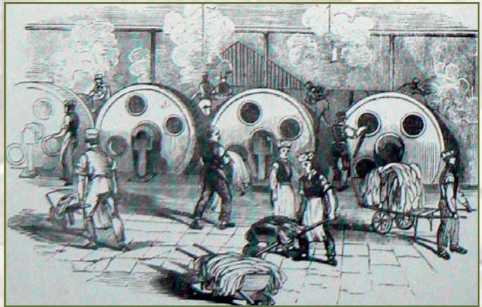
Dash wheels at Thomas Hoyle's bleach works in Dukinfield captured on a print of 1843
