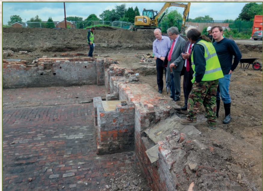
Salford City Councillors viewing the excavated remains of Pendleton Old Hall (© GMAAS)
