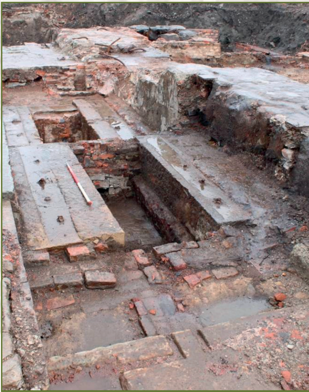
Foundation beds for the main steam engine
