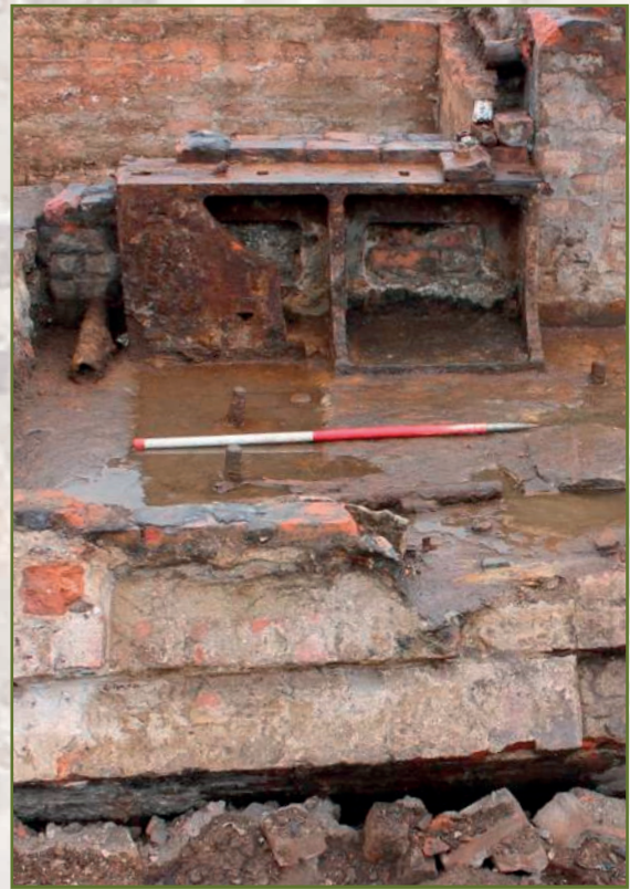
Iron casting that housed the transmission gearing
