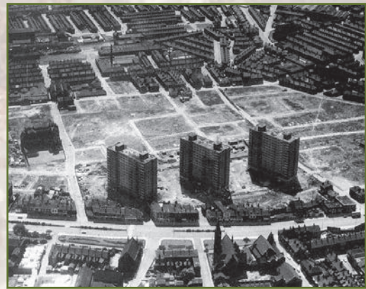
The first three residential towers to be built in Pendleton in the early 1960s (© University of Salford)
