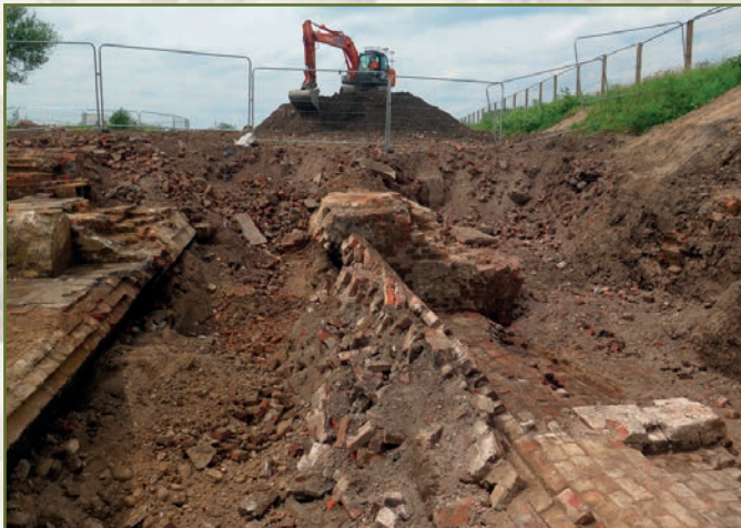
The base of the vaulted capping during excavation (© Salford Archaeology)
