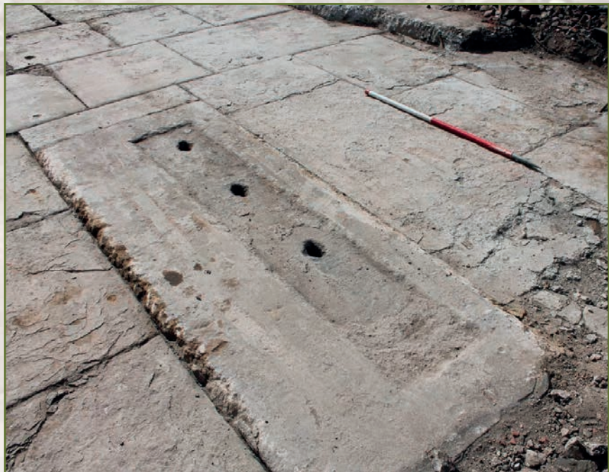
One of the stone machine bases set into the flagstone floor of the bleach croft
